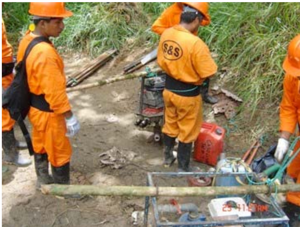
Fig. 11 – Drilling crew preparing to move portable drill
